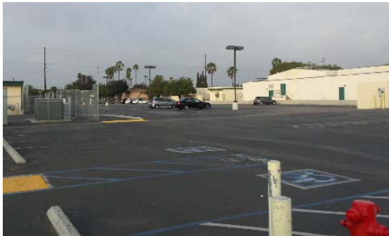
Parking lot is in need of renovation and improved traffic flow.
