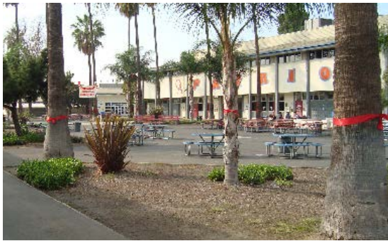
Central quad in poor condition.
