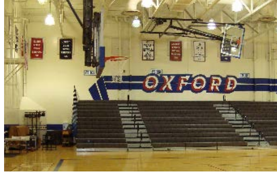
Gym is in need of a lobby with restrooms.
