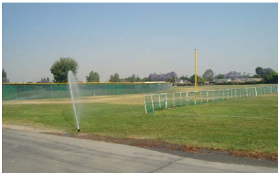
The athletic fields need new irrigation system.
