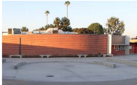
Loara Theater in need of upgrades.
