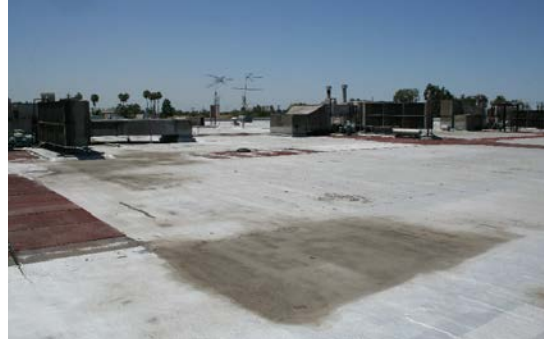
Replace roofing and HVAC units.
