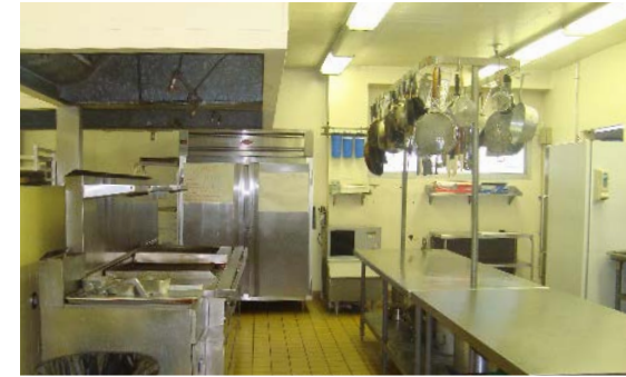
The central kitchen is undersized and needs major renovation.
