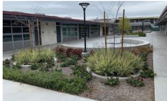
Completed - Courtyard Modernization
