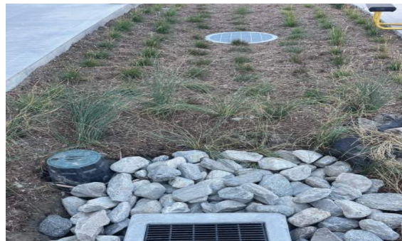
In Progress - Bioswale
