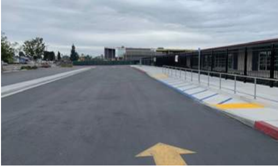
Completed - Drop-Off Parking
