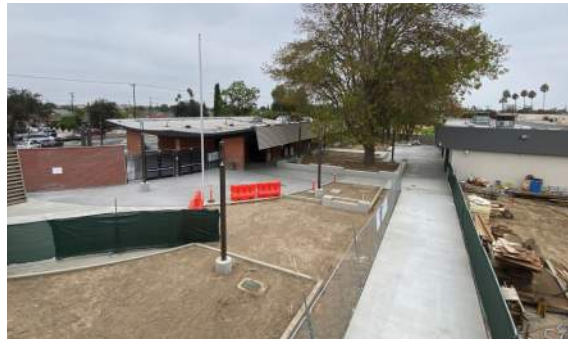
In Progress - Site Work
