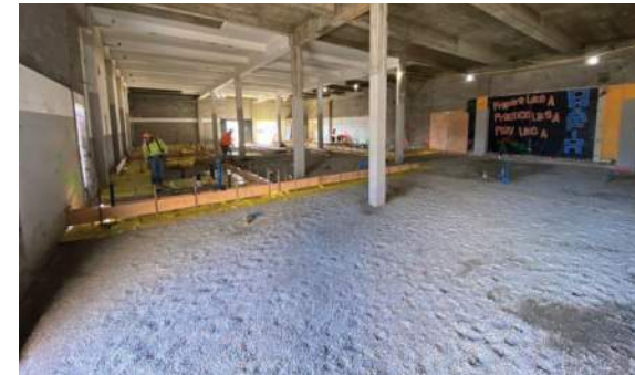
In Progress - Shower/Locker Room
