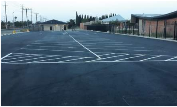
Completed - Main Parking Lot
