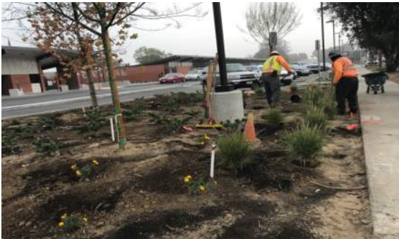
In Progress - Drop-Off Loop Landscaping
