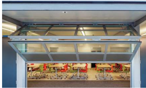
Completed - Bldg. 2 & 4 Modernization
