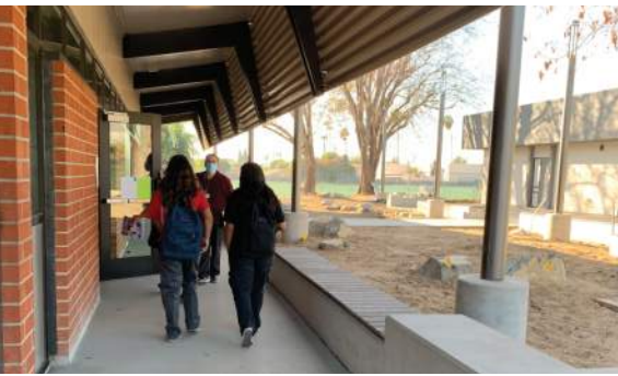
Classroom Courtyard & Walkway
