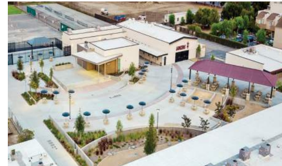
Completed - New Quad Modernization
