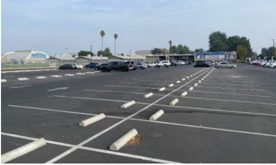
Main Parking Lot
