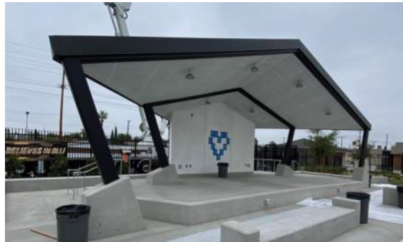
Completed - Stage Structure
