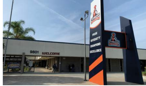
Front Entry & Marquee
