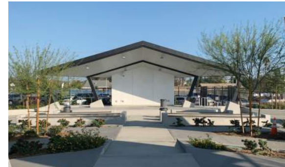
Completed - Stage Structure
