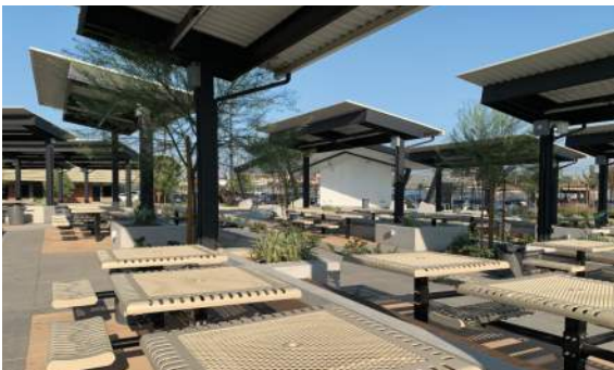
Completed - Benches, Tables, Shade Structures
