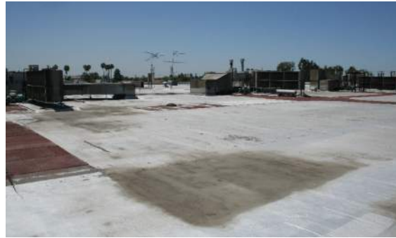
Replace roofing and HVAC units.
