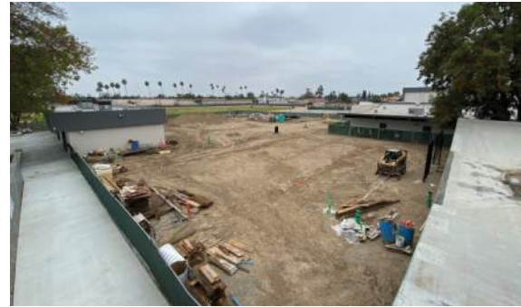
In Progress - Buccy Cove
