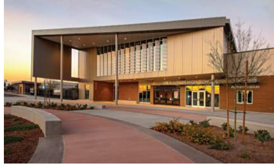
Completed - New Two-Story Building
