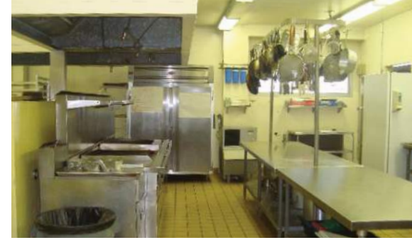
The central kitchen is undersized and needs major renovation.
